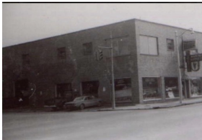
From the Bowling Green Univ. archives. A view of 1 South Summit Street on the Maumee River, the 1939 location of Bodette Marine.
